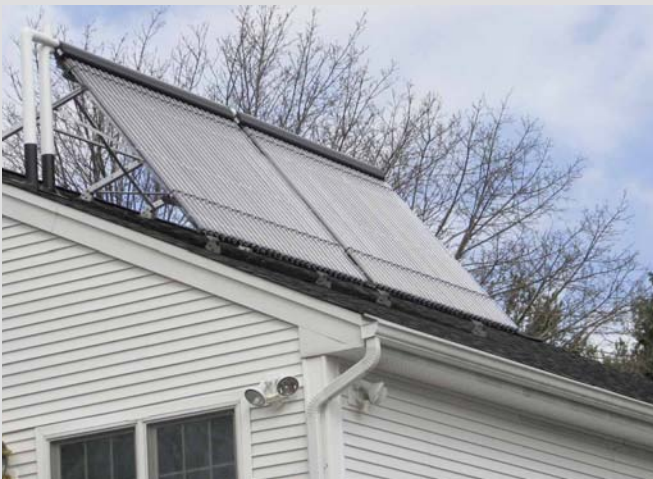
Vitosol 300 – vacuum tube solar collectors
