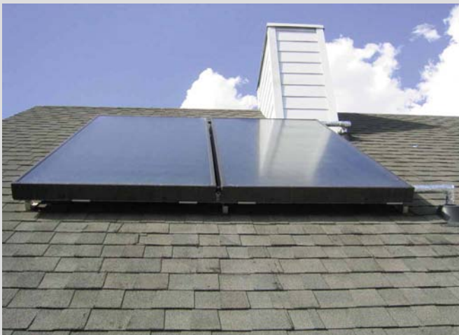
Vitosol 100 – flat plate solar collectors
